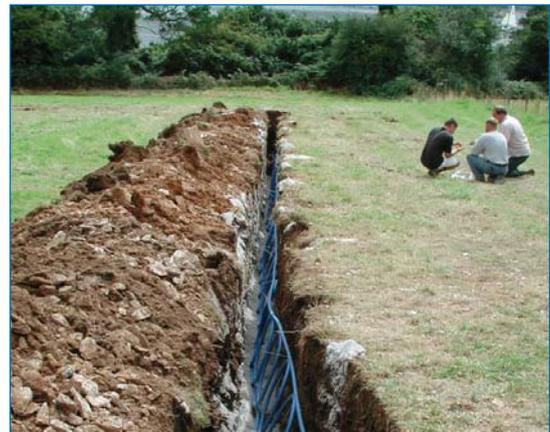
Figure 7: Ground loop and trench for ground source heat pump
