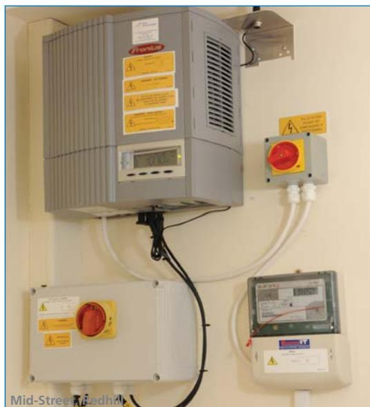
Figure 2: Photovoltaic inverter
